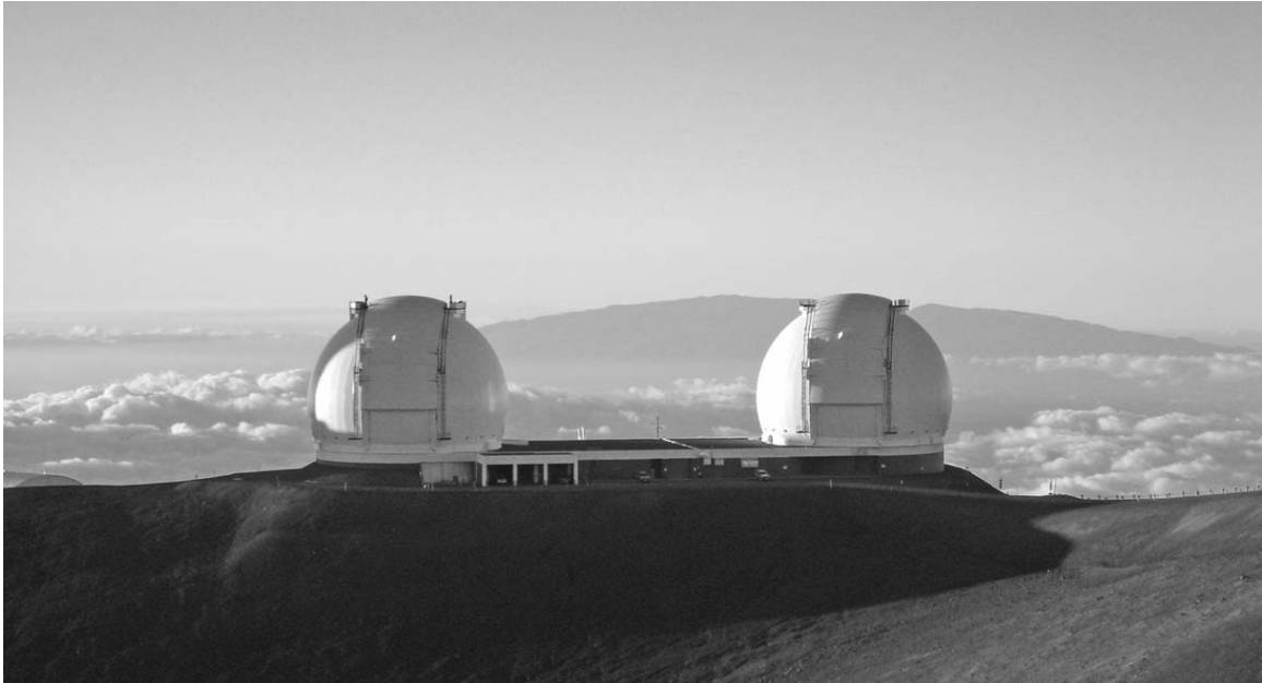
Fig. 3.2 The twin domes of the W.M. Keck Observatory on the summit of Mauna Kea. Each dome encloses a telescope with a segmented mirror having an effective aperture of about 10 meters. The domes are 85 m apart.
